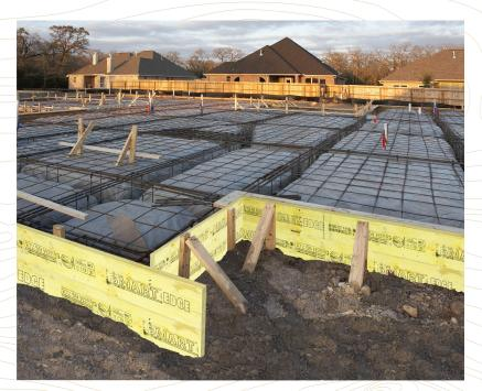
SmartEdge is a lightweight LVL, engineered wood product utilised in concrete construction applications.
