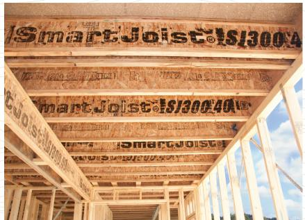
SmartJoist is an Engineered Wood I-Joist manufactured with LVL flanges top and bottom, joined with an OSB web.
